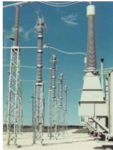
Figure 6. 500kV MOSAs at Manitoba Hydro AC-DC converter stations (1979)
