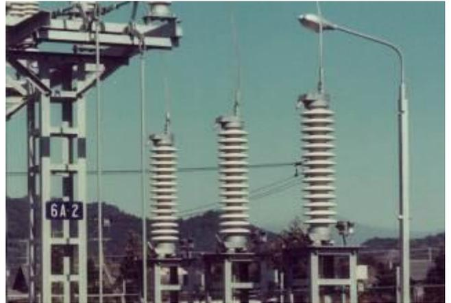
Figure 4. MOSAs at Hayato SS of Kyushu Power Co.: 66kV heavy pollution type (0.12 mg/mm<sup>2</sup>) (1975)
