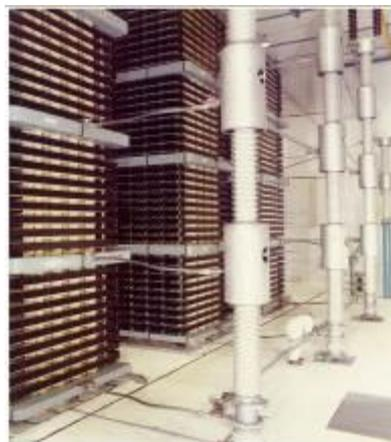
Figure 8. MOSAs in Dover Channel converter station (1984)
