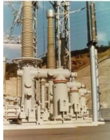
Figure 5. 500kV MOSAs for GIS of Kyushu Electric Power Co. (1975)
