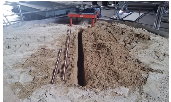
Figure 15. Photograph of copper pipes used to simulate ground electrodes.
