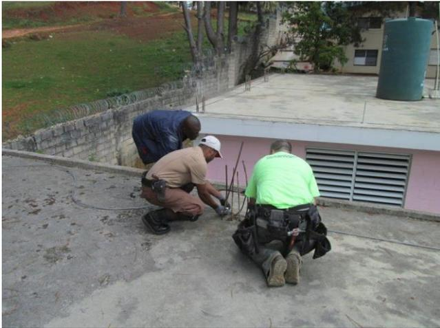
Figure 2. Installers making interconnection with reinforcing steel for use as air termination with completed structure in background
