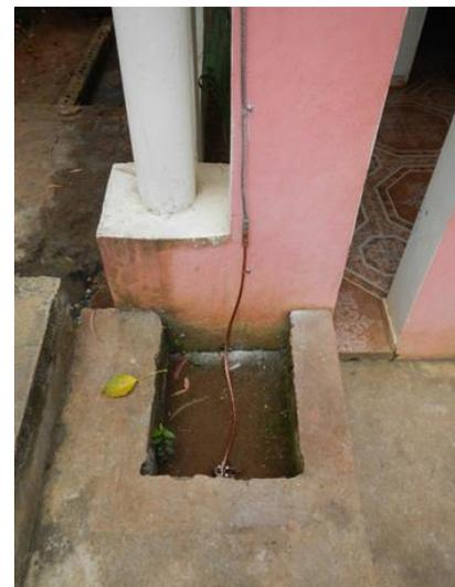
Figure 3. Earthing electrode showing aluminum to copper transition at down conductor
