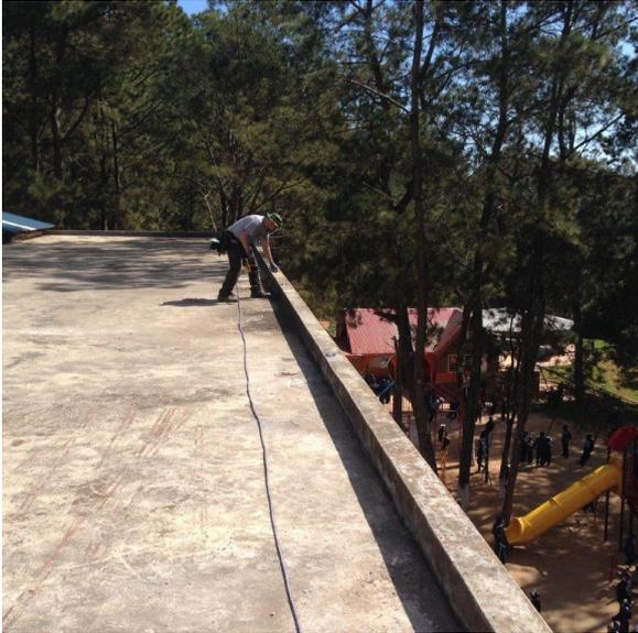
Figure 4. Installation of air terminal base on parapet wall on primary school
