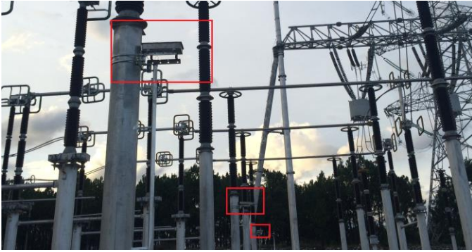
Figure 9. Location of the sensor in practice
