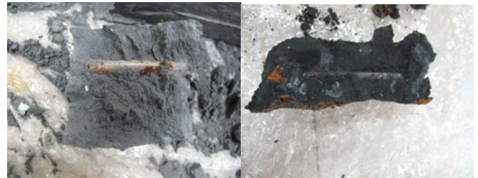
Figure 5. Corrosion of Samples in Earthing Enhancing Compound
