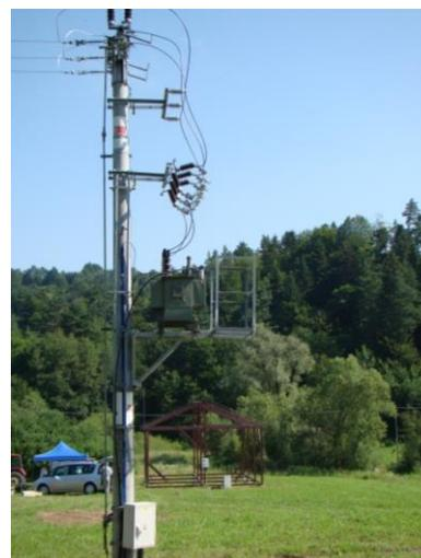
Figure 1. Test site in Huta Poreby, Poland equipped with a test house connected to the transformer station and the 500 m long overhead power line.
