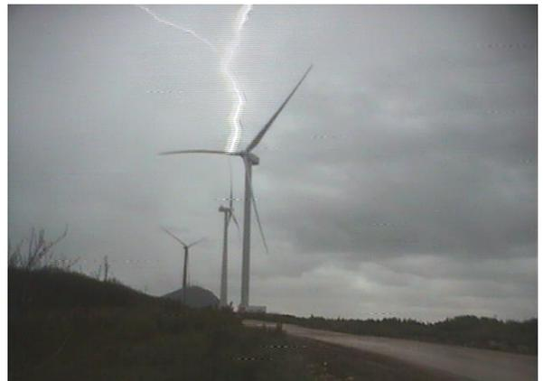
Figure 9. Upward lightning from the tip of the central wind turbine analyzed by Author [11]. The flash was not detected by LLS which has a peak threshold of 2.3 kA.
