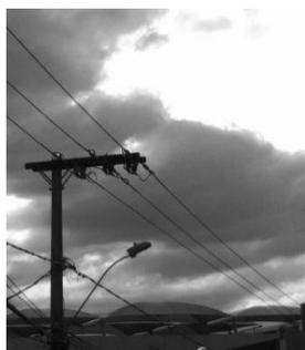
(a) Conventional configuration with bare conductors.
