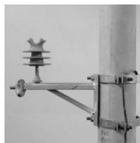
(a) Pin type polymeric insulator.
