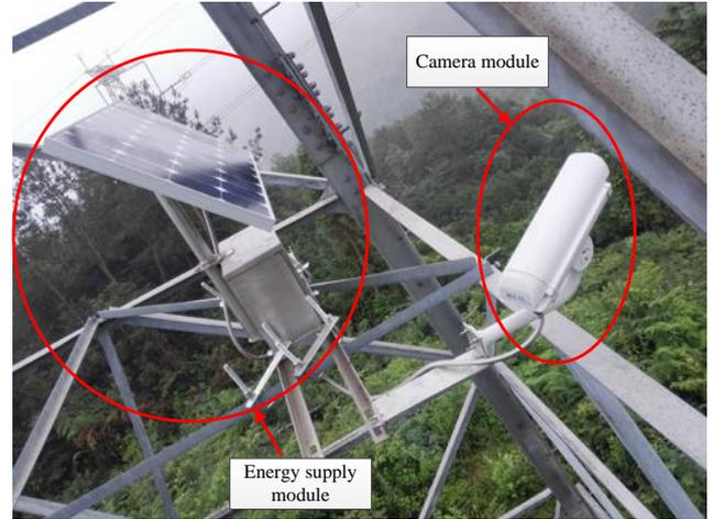
Figure. 2 Monitoring terminal is usually installed on the tower of the 500kV transmission line
