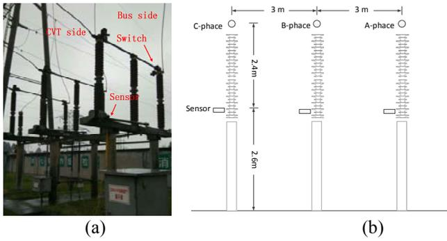
Fig. 7 Placement of the sensors in the substation
