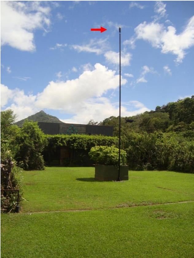
Figure-3: The lightning protection system intended to cover an open roof-top terrace in a hotel in Sri Lanka. The red arrow indicates the ESE type finial on the supporting structure.
