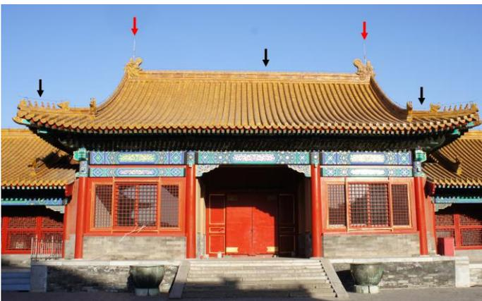
Figure-4: The lightning protection system of a low-rise building with archaeological value, in Beijing China. Black arrows show the continuous air-termination system (an aluminium conductor with circular cross section) and red arrows show the ESE air-terminations.
