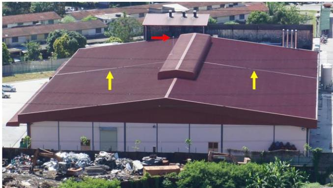
Figure-5: An all-metal structure used as a machinery store house in Malaysia. The red arrow indicates the ESE type finial on the roof and the yellow arrows show the copper down conductors painted white
