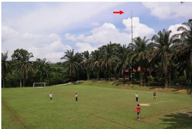
Figure-1: The lightning protection system intended to cover a playground of a school in Malaysia. The red arrow indicates the ESE type finial on the tall supporting structure.
