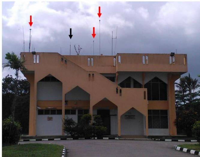
Figure-6: An observatory building in Johor Bharu, Malaysia. The red arrow indicates the ESE type finial on the roof and the black arrow shows the conventional air-termination.
