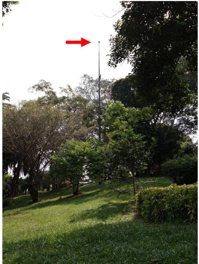
Figure-2: The lightning protection system intended to cover an open hill-slope of a school in Malaysia. The red arrow indicates the ESE type finial on the tall supporting structure.
